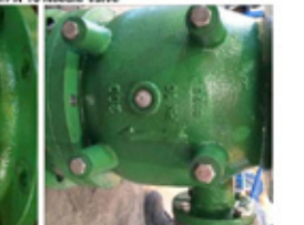
Fig. 17 & 18- DN 200/PN 10 Needle Valve Marking
