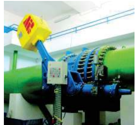
Normally open (fail to close) emergency Excess shut-off valve DN1800, PN25 Water supply project in Algeria, Contractor: Efacec (Portuguese corporation)
